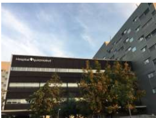
Figure 2a) Hospital Quironsalud Barcelona
